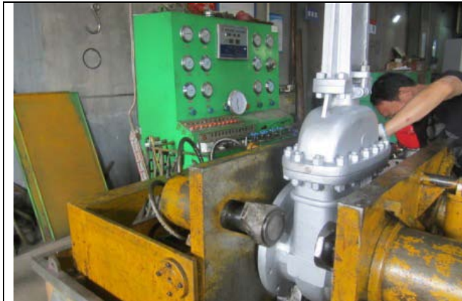
Pressure test is ongoing
