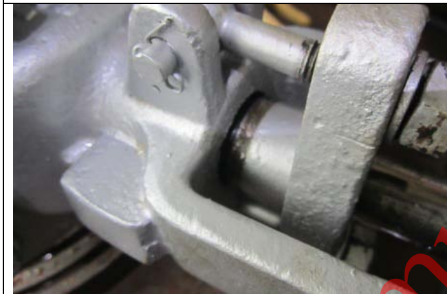
Packing gland is loosened for backseat test
