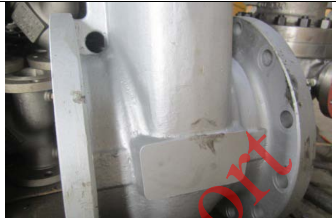
Dirt, oil stain and local paint damage caused by pressure test to be repaired
