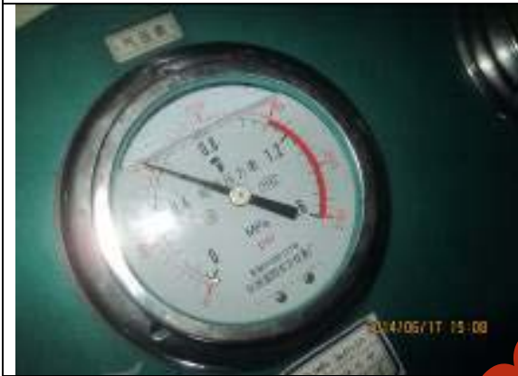
Showing the air closure test.
