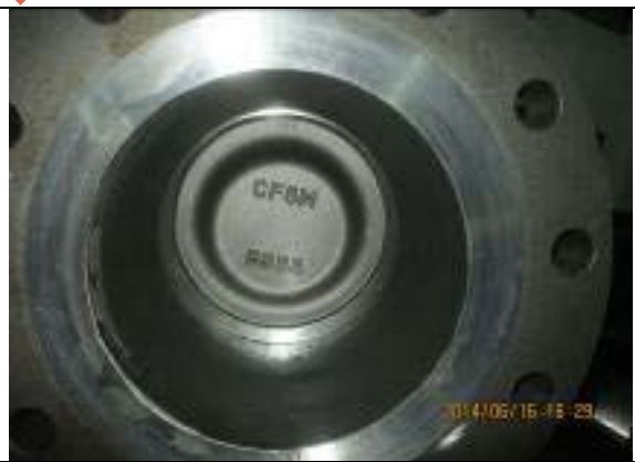
Checking leak during high seat closure tests.
