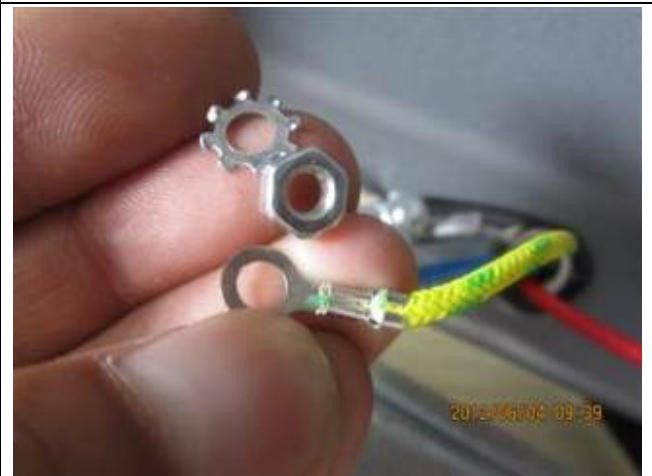
The earth connection
